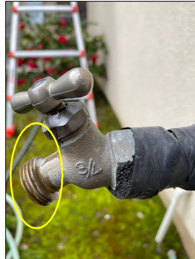
No pressure relief valve on all outdoor spigots.
