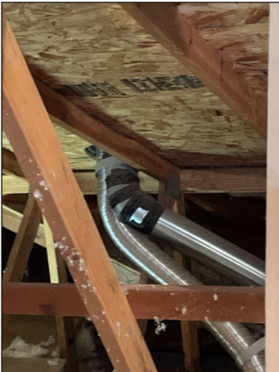
Incorrect taping material utilized to join vent connections for dryer vent. Recommend removal of tape and correct joining of vent piping.
