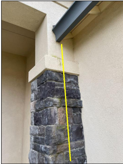
Leaking gutter
