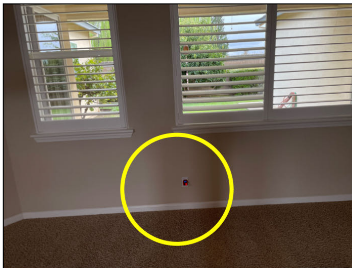
Open Ground showing only on the top portion of the receptacle underneath the window in the living room.
