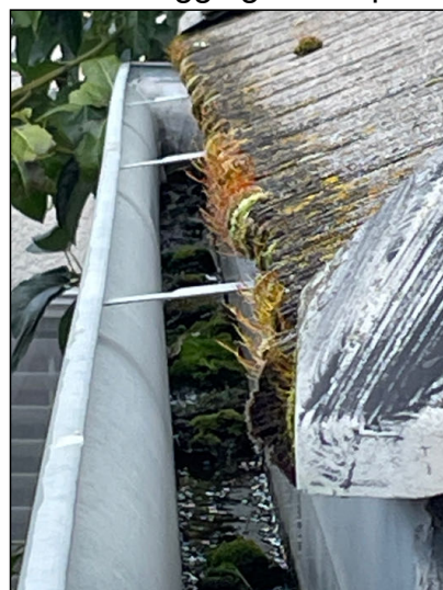
Debris clogging downspout
