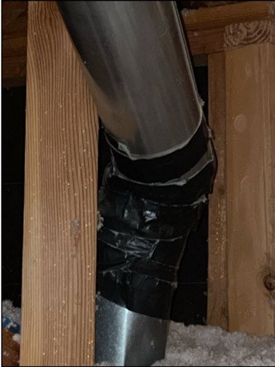
Incorrect taping material utilized to join vent connections for dryer vent. Recommend removal of tape and correct joining of vent piping.
