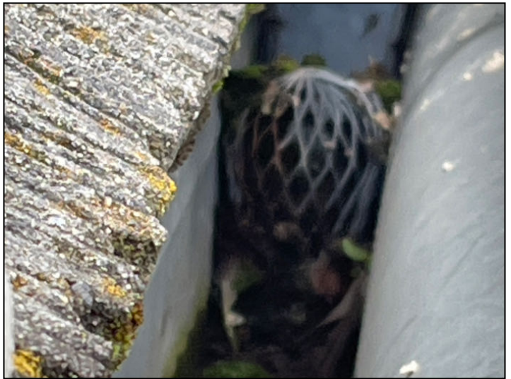
Debris clogging downspout
