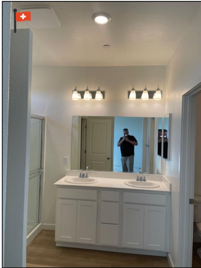
MBR Bathroom. See additional photo and caption regarding incorrect placement of receptacle near the shower.
