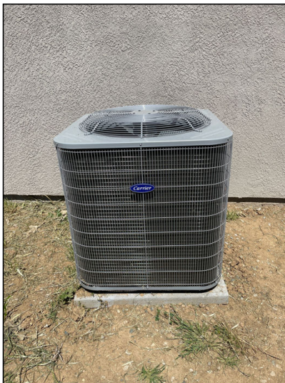
Carrier AC condenser unit and heat pump system.
